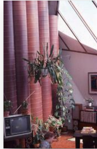
Tall containers of water serve as thermal mass heat storage in this open design solar home.
