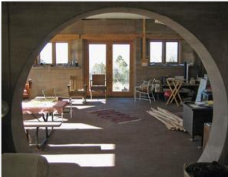
Thermal mass can be used in innovative ways – rammed earth interior wall molded into an attractive arch doorway.
