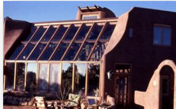
The south side opens up to the sun in this Sunspace passive solar design.
